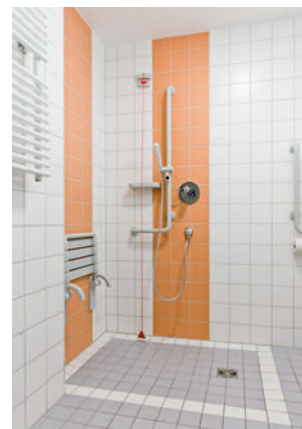
Fig 2.5-8 Patient bathroom with barrier-free access to the shower and handlebars with fold-out seating.
